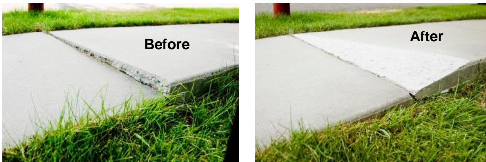
Figure 7: Precision Sidewalk Safety Work Example
